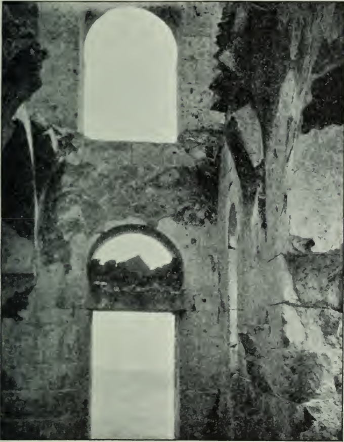
FIG. 336.—Tchangli Klisse, interior of narthex, looking S.
